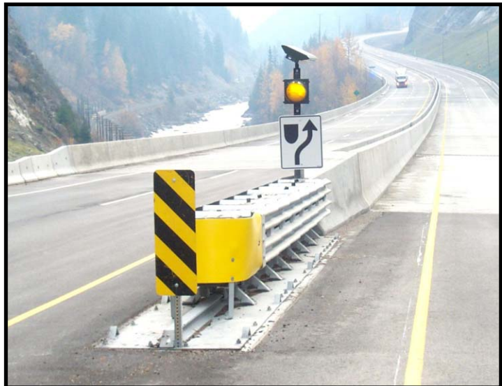
R247 24 Hour Flasher installed on Canada's Transcanada Highway as part of the Yoho Bridge Project. Photo submitted November 10, 2004, by Peter Kiewit Sons', Inc.
